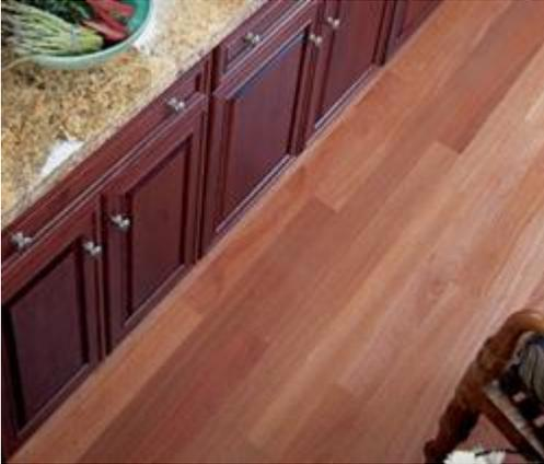
Figure 5: Feature veneer plywood overlay flooring
